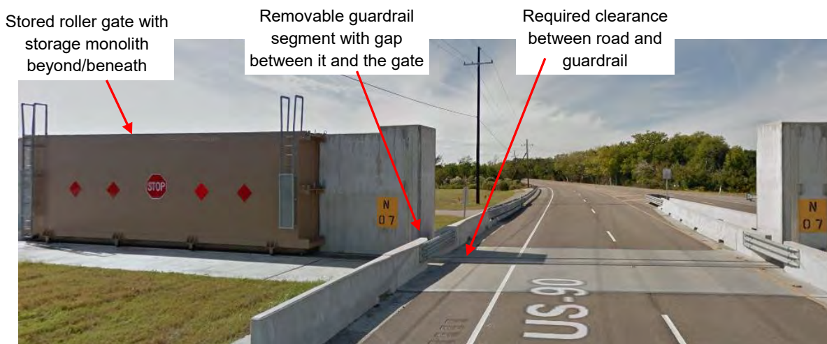
Figure 7.2 – Roller Gate with Removable Guardrail Arrangement
