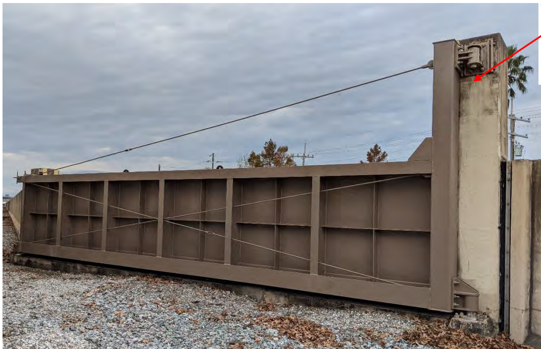
Figure 7.3 – Swing Gate with Large Length-to-Height Ratio
